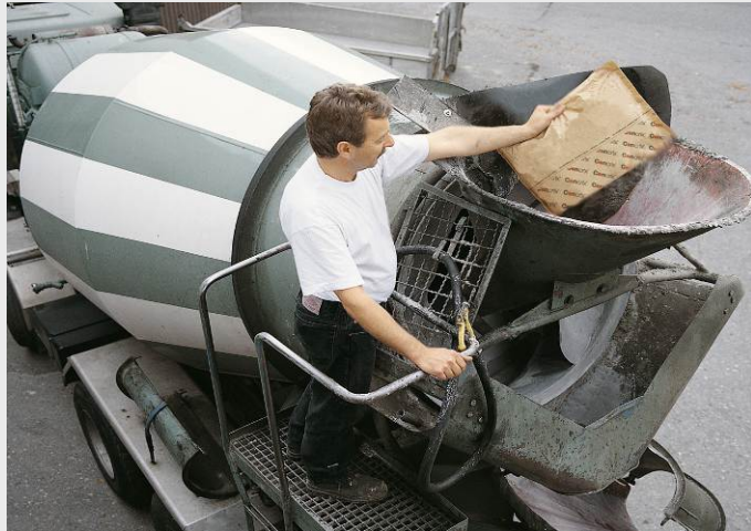
Adding directly to mobile concrete mixer
