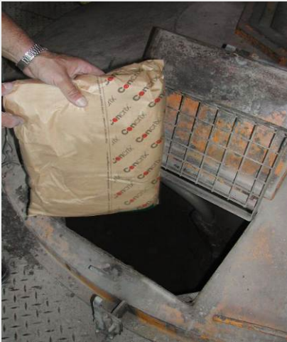
Adding in concrete production facility
